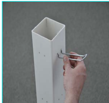
Step 4- Attach post hangers (5)
